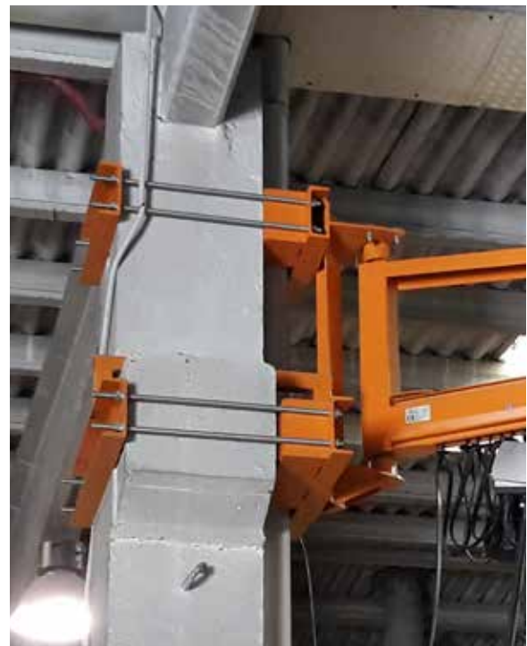
CONCRETE COLUMN BRACKETS
