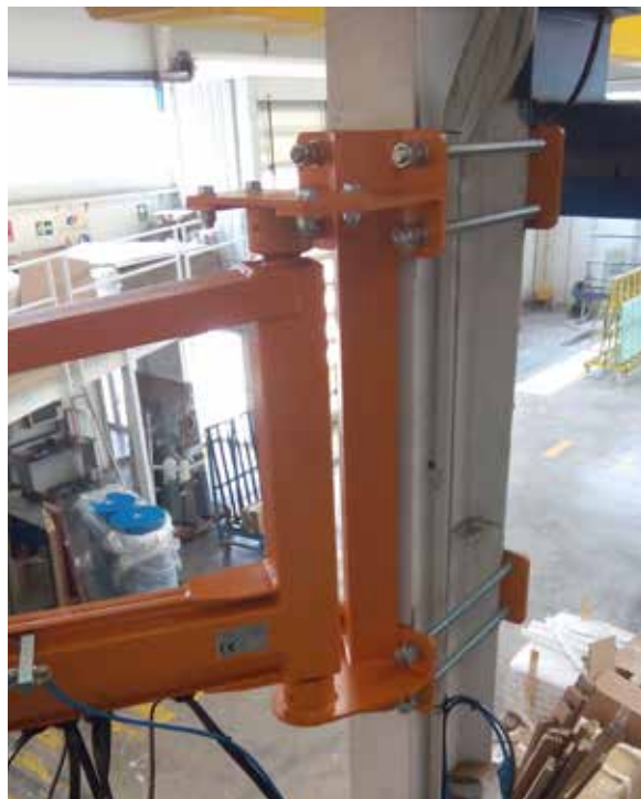
METAL COLUMN WELDING + REINFORCED BRACKETS
